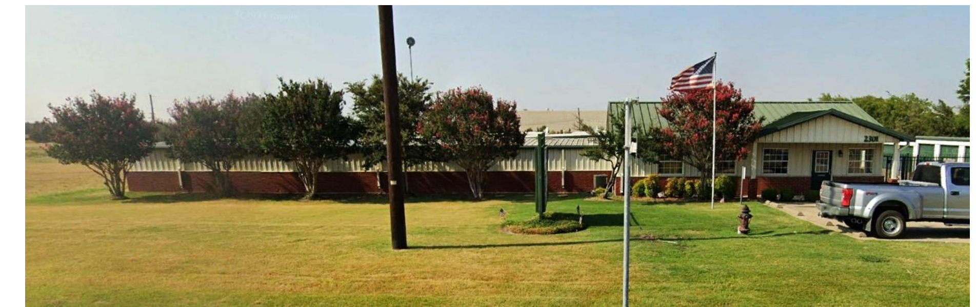
EXISTING HIGHWAY 276 FACADE
